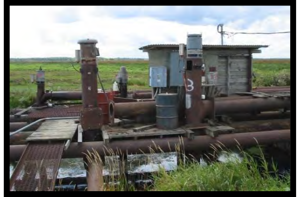
Typical pumping station
