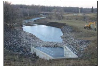
Looking downstream from outlet structure
