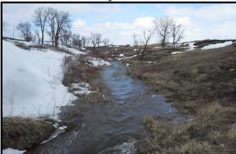
Rapidly flowing runoff in Polk County Ditch 1. A lot of bank failure and sloughing is occurring along the channel.
