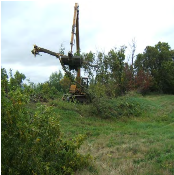
Clearing trees to get at the ditch
