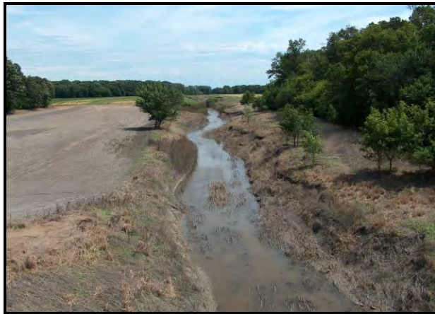
Looking East before construction (CSAH #64)
