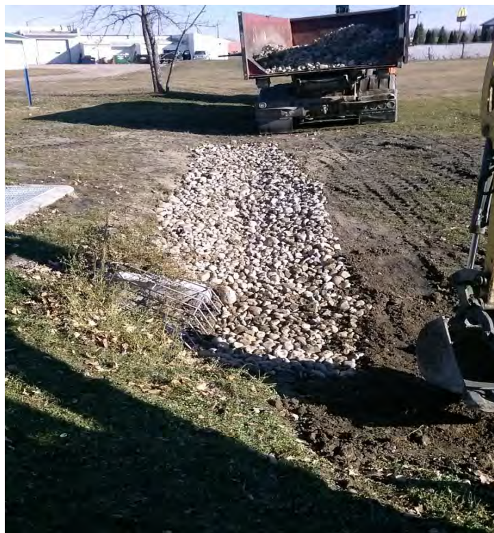
Reierson Construction with completed rock erosion site
