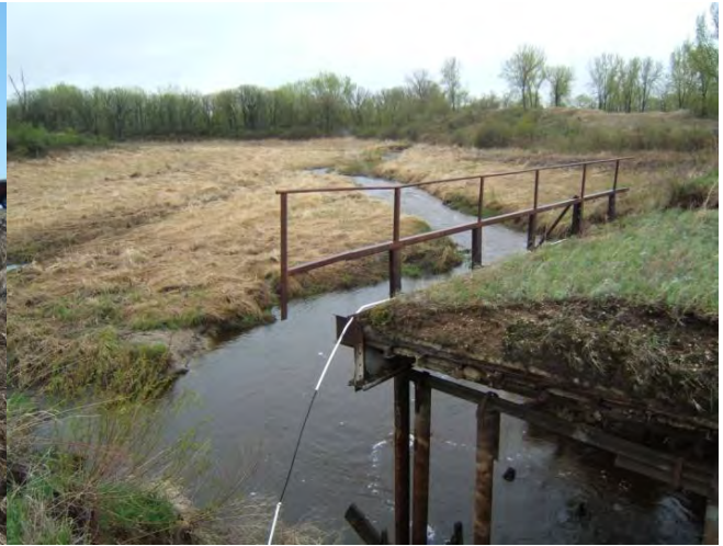
Washed out old bridge will be removed
