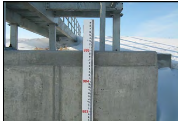
Typical staff gage at structure
