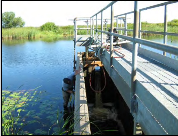
Installing staff gauge – Moose R. Impoundment
