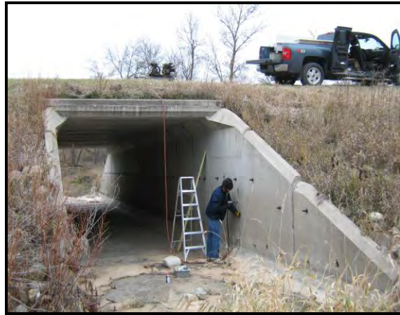
Installing staff gauge Browns Creek, Red Lake Co.
