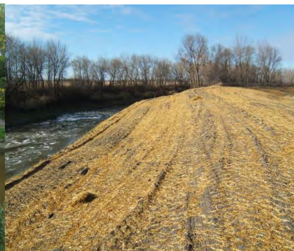
Spoil pile after cleaning seeded and mulched
