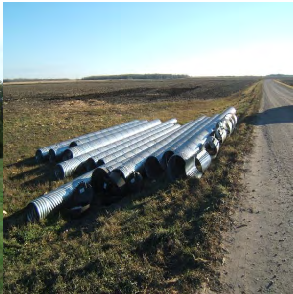
Load of pipe and traps for Ditch 83
