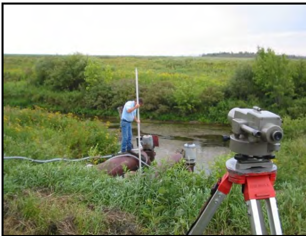
Surveying water lift from river to pump
