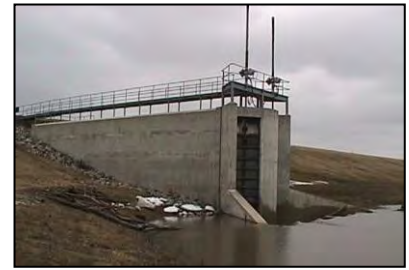
Principal outlet structure hydraulic gate operation
