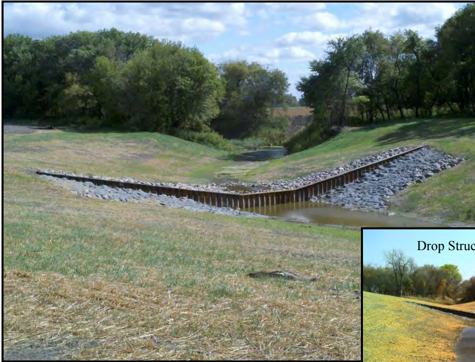
Drop Structure at Station 15+50
