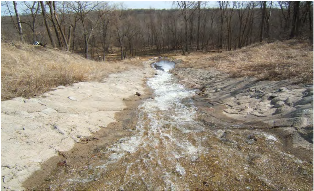
Runoff water flowing in the rock chute on RLWD Ditch 10 (Project #161)
