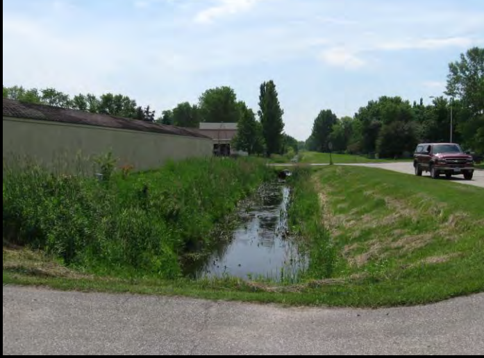
Edgewood Drive before Construction
